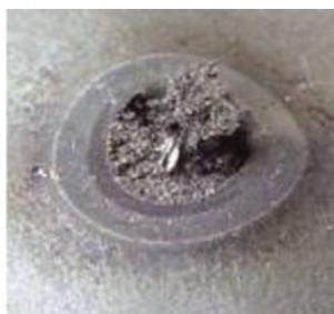
Interfacial Fracture with Partial Thickness Fracture
