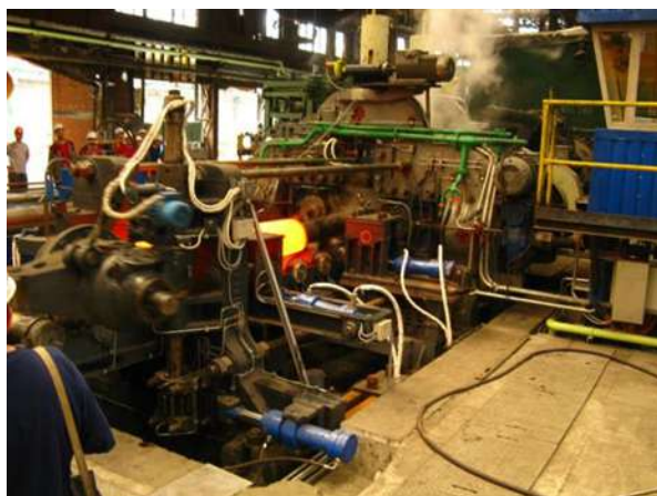
Fig. 14.26 Piercing mill – front view
