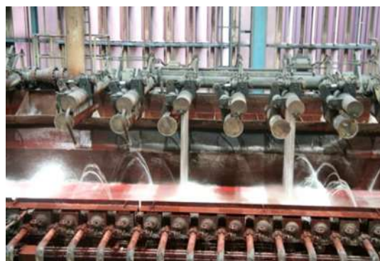
Water cooling - detail
