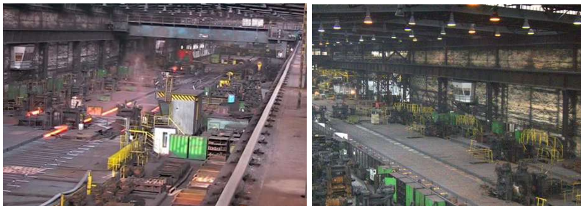
Fig. 7.5 View of cross-country arrangement of roll stands in rolling mill HCC
