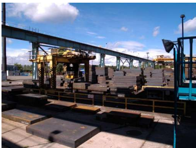
Fig. 5.4 Slab storage yard
