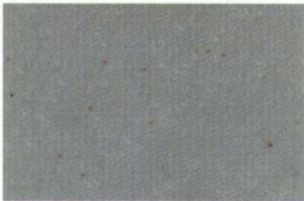
Rust Grade 9-P, 0.03% Rusted
