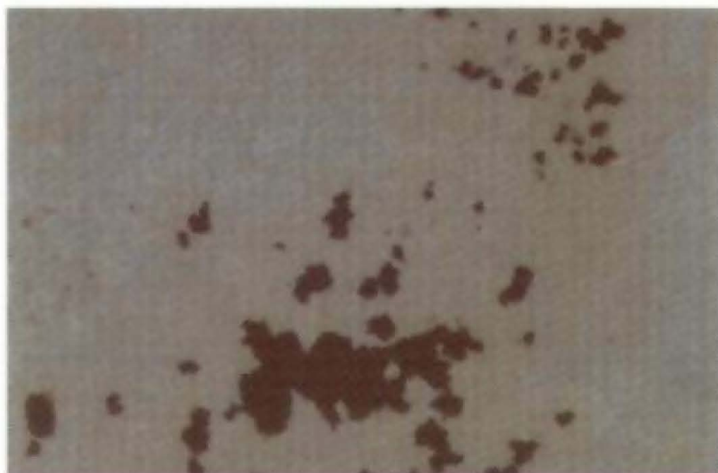
Rust Grade 4-G, 10% Rusted
