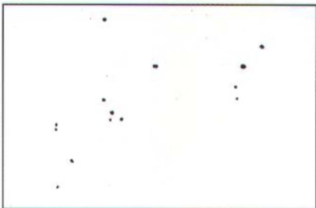
Rust Grade 8-G, 0.1% Rusted
