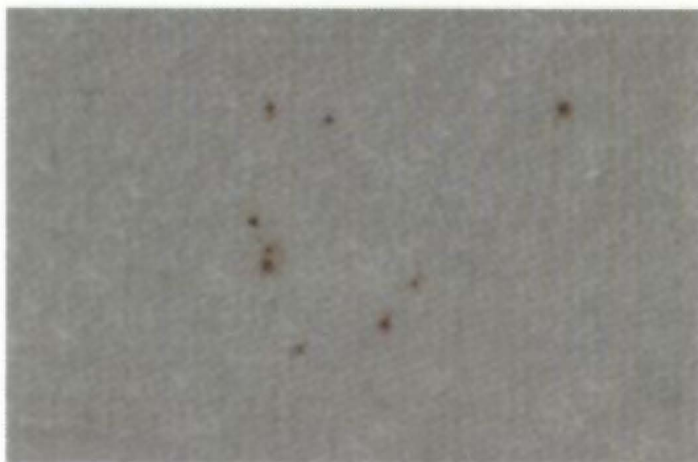
Rust Grade 9-G, 0.03% Rusted
