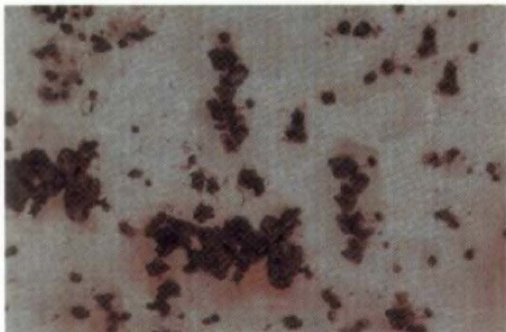
Rust Grade 3-G, 16% Rusted
