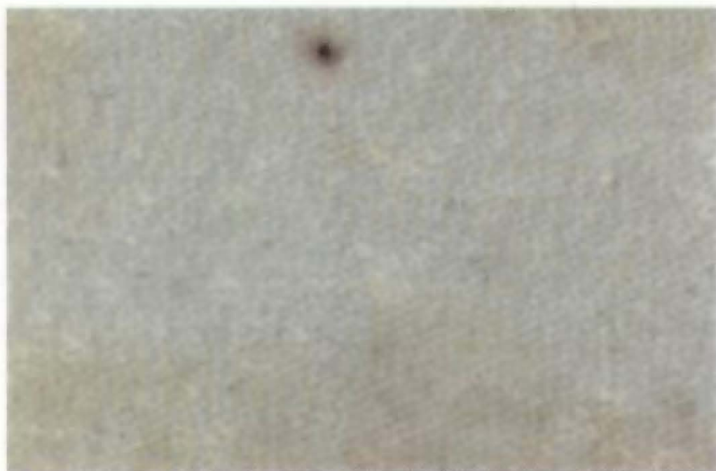
Rust Grade 9-S, 0.03% Rusted
