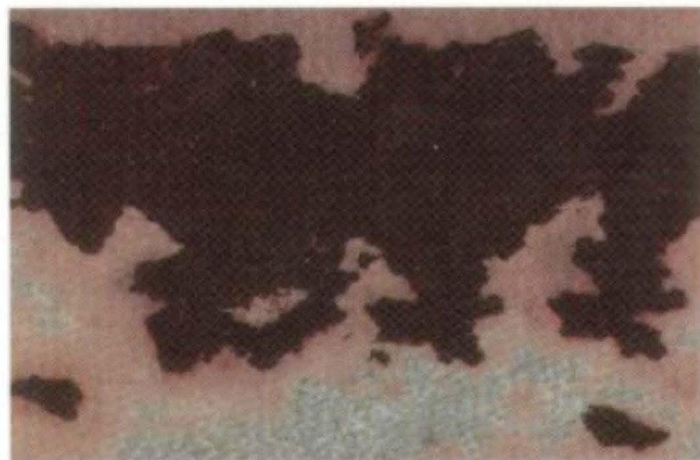
Rust Grade 1-G, 50% Rusted
