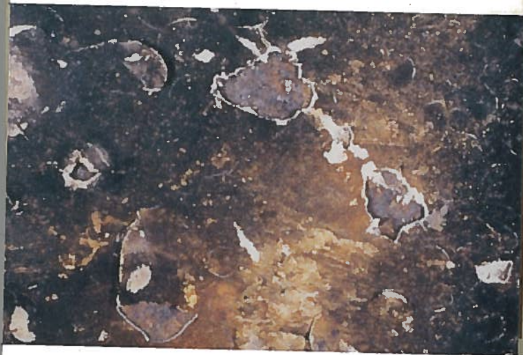
INITIAL CONDITION H
