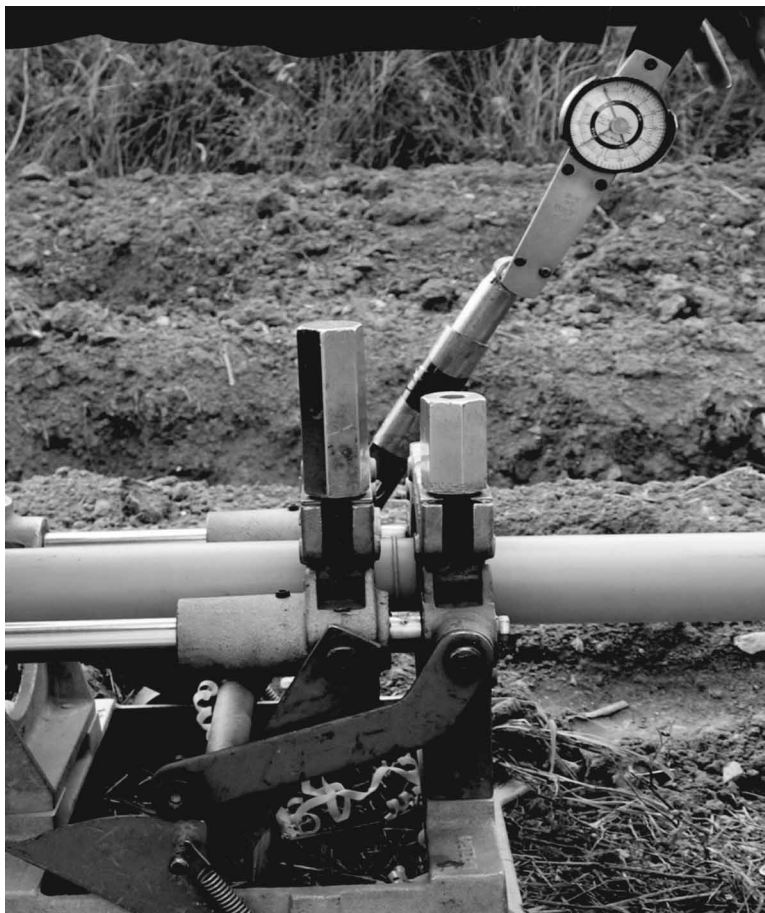
FIG. 7—Butt fusion of PA-11 piping using standard PE butt fusion equipment.
