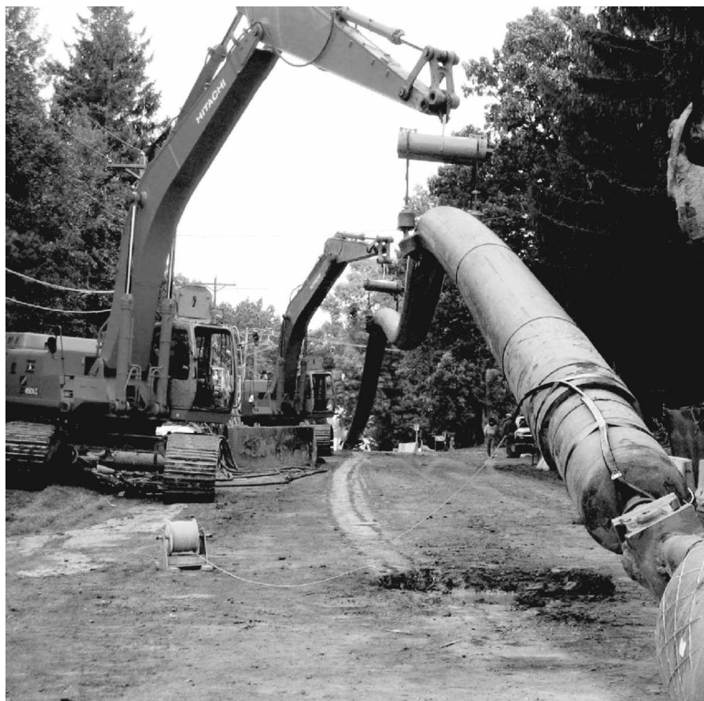
FIG. 1—HDPE pipe at White Bear Lake, MN.
