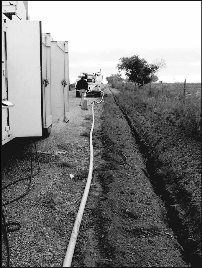
FIG. 2—Coiled PA-11 pipe after straightening, ready to be rolled into the trench.
