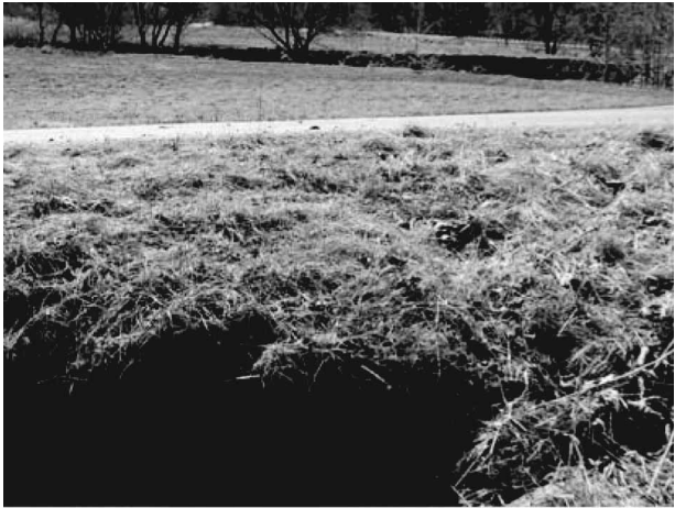
FIG. 1—Ohio DOT Installation of 24 in. (600 mm) diameter culvert after 27 years in acid mine run-off.
