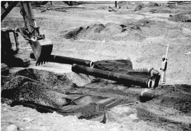
FIG. 4—From FEMA P-675, installation of profile wall corrugated pipe for a drainpipe replacement during a modification of an embankment dam [25]. Corrugated polyethylene pipe has been used successfully to reline failing pipe by a number of agencies. In 1983-84, the Oklahoma Department of Transportation relined over 40 corroded steel pipe crossdrains. In 2007, the Delaware Department of Transportation relined a failing reinforced concrete pipe under a major thoroughfare in Wilmington, DE, with no disruption of traffic and an estimated savings of nearly $1 000 000 versus removing and replacing the existing pipe.
