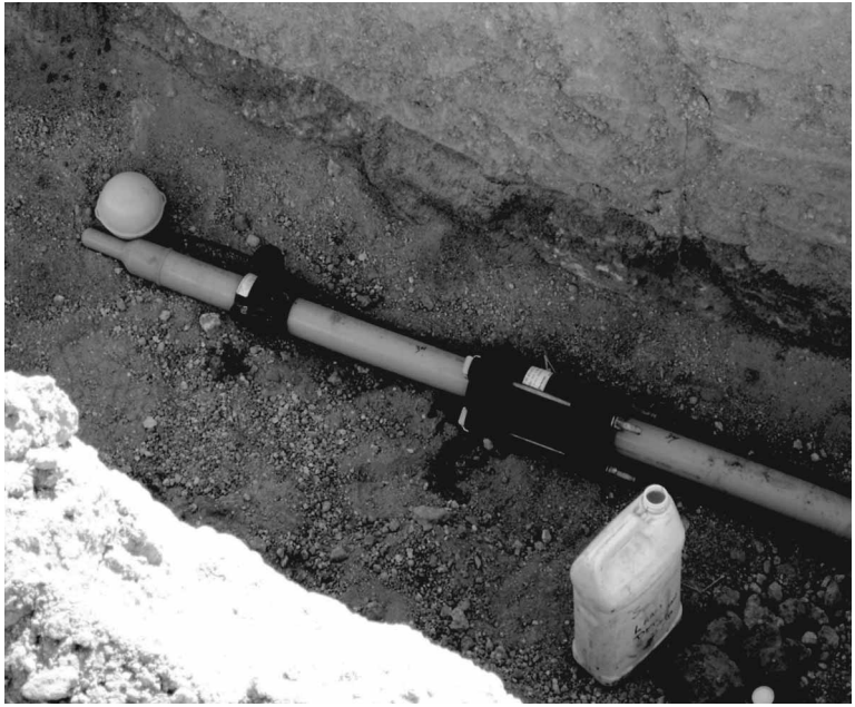
FIG. 11—Using mechanical couplings and tapping tees on PA-11 gas piping.
