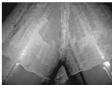
8d, Extrusion welding. (This fitting has been prepared for fiberglassing in the area near the extrusion weld.)
