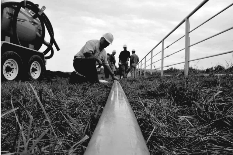
FIG. 1—High pressure PA-11 piping ready for installation.
