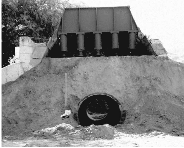
FIG. 2—Utah State University: soil cell full, loading beams down, and load being applied to soil surface over 60 in. (1500 mm) pipe.
