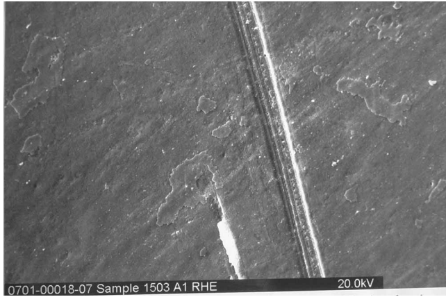
FIG. 3—Flaking and crack in CPVC pipe having mixed glycols in sprinkler system.
