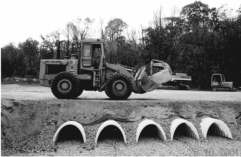
FIG. 5—Live load testing of 30×51 chamber.
