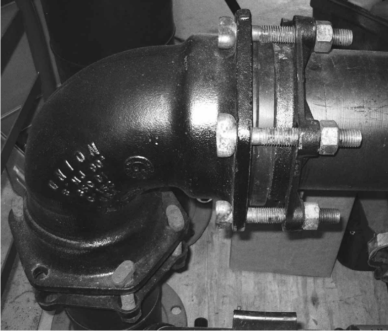
FIG. 3—HDPE MJ adapter (on right) and DI elbow.
