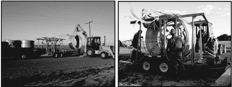
FIG. 3—Loading 1000 ft coils of PA-11 Pipe onto installation trailer.
