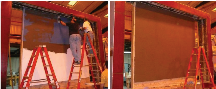
FIG. 17 Installation of basecoat and mesh over encapsulated VIP panels.
