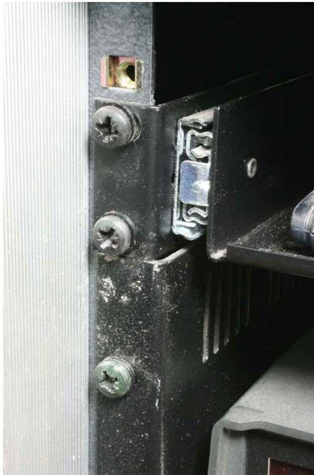
Fig. 8-8: Equipment secured using rack nuts and screws.
