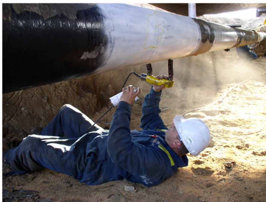
Figure 8.1: Bottom of pipe In-the ditch SCC assessment using BWMPI technique
