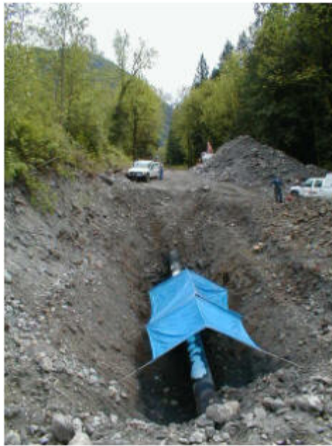
Figure 5.3: SCC site investigative dig
