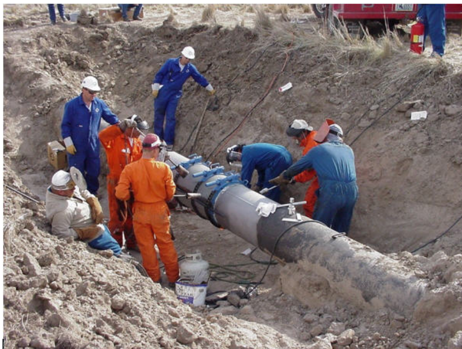
Figure 9.7: Steel Reinforcing Sleeve
