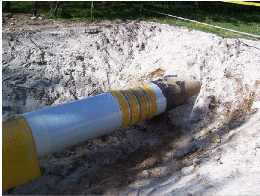
Figure 9.9: Composite reinforcement sleeve repair
