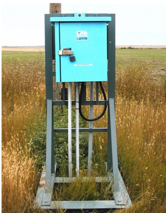
Figure 9.3: CP rectifier
