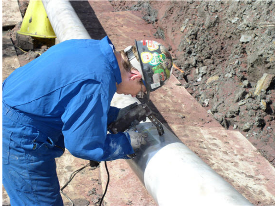
Figure 8.2: Top of pipe in-the ditch SCC assessment using BWMPI technique
