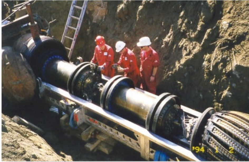
Figure 6.4: Shear wave ultrasonic tool being retrieved from temporary receiver barrel
