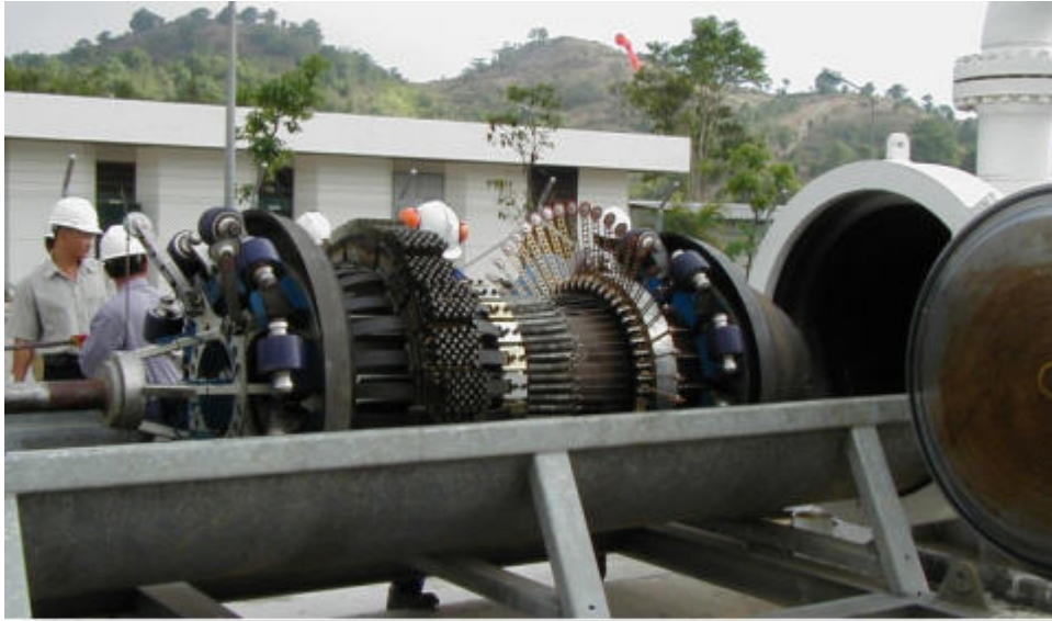
Figure 6.1: In-line inspection tool being loaded into a 'pig launching barrel'
