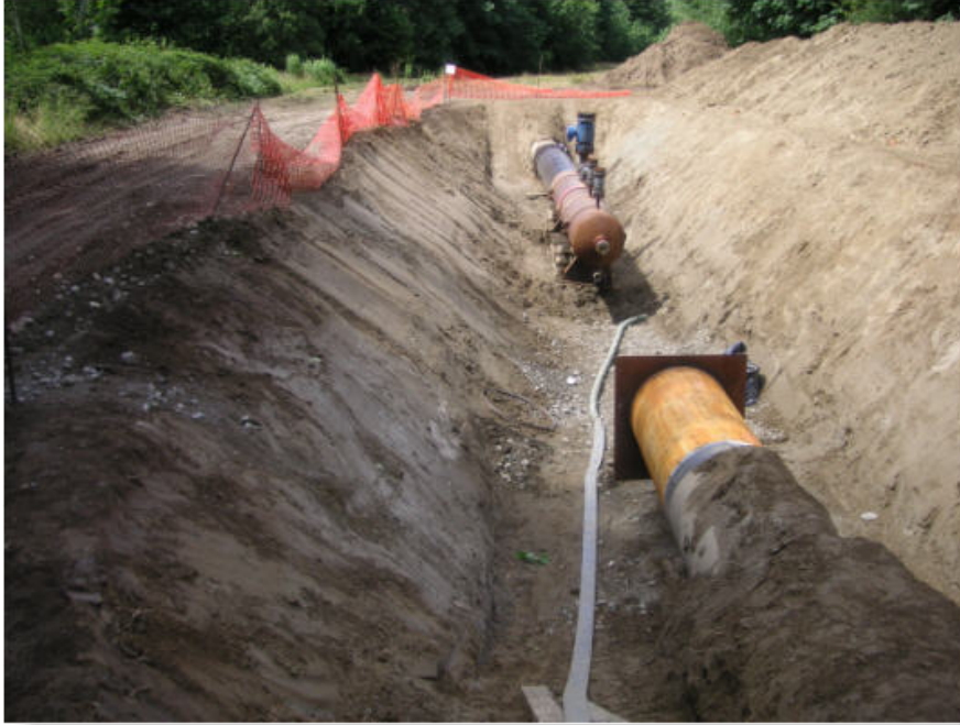
Figure 9.4: Hydrotest 'test head' and manifold set-up
