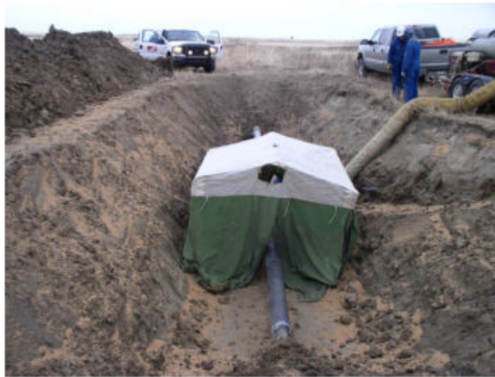
Figure 9.2: Hording-In an Excavation Site for Winter Recoating
