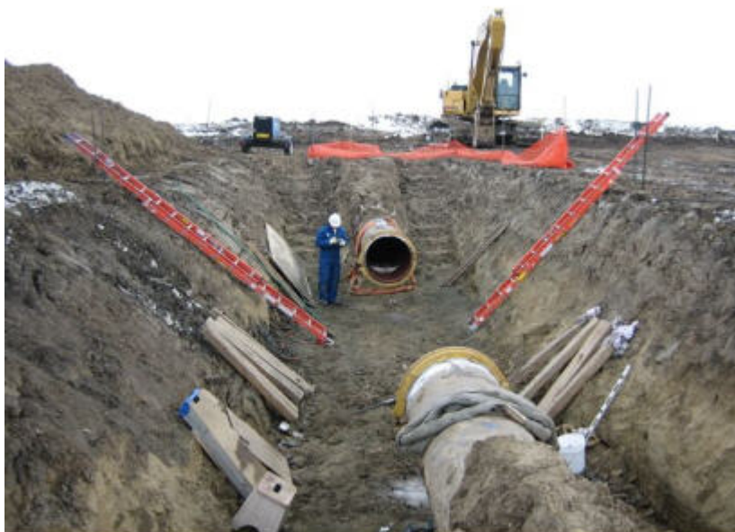
Figure 9.11: Repair by pipe replacement
