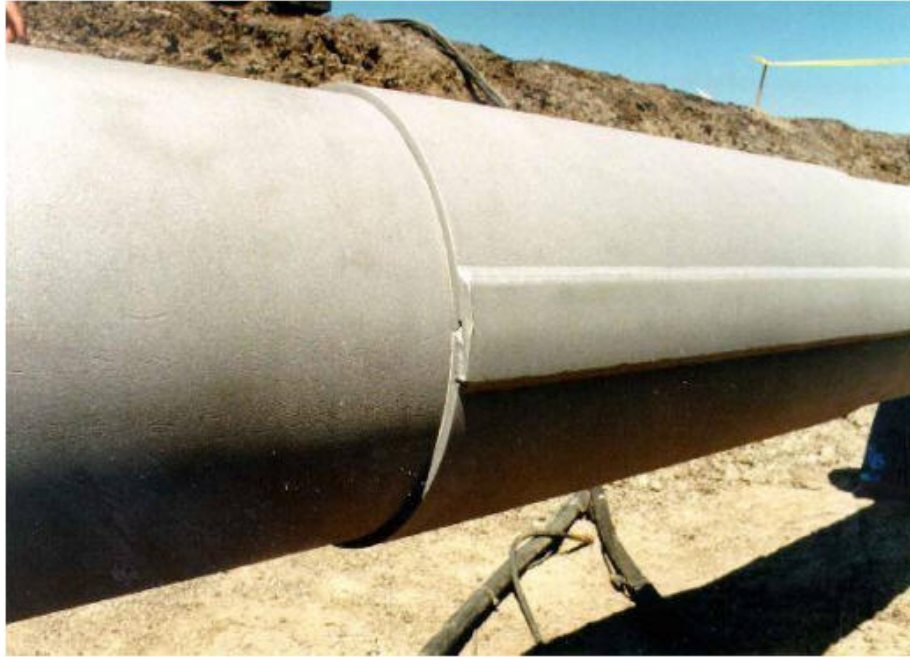
Figure 9.7: Steel Reinforcing Sleeve
