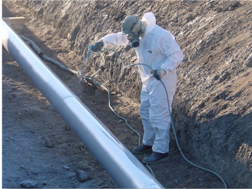
Figure 9.1: Application of Liquid Based Coating after Bell Hole Inspection
