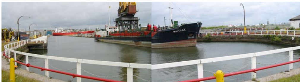
Bidston Dry Dock – 8m depth used for submerged mid-scale tests.
