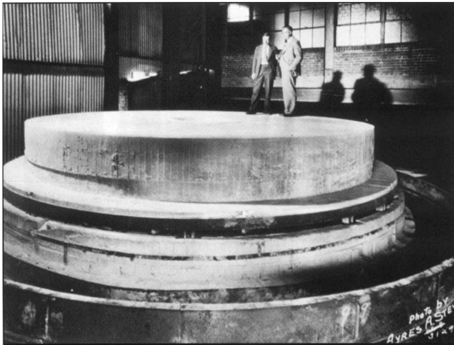
Figure 5-22. 200 inch mirror blank ready for shipping by rail from Corning, NY, to Pasadena, CA. (Photo courtesy of the Corning Incorporated Department of Archives and Records Management, Corning, NY.)
