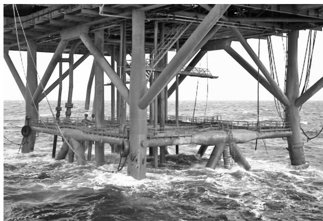
Figure 1.3 Typical design of a fixed offshore structure, such as the base for an offshore oil or gas platform in the North Sea (© TWI).
