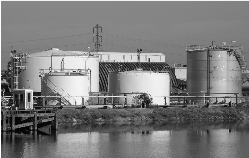
Figure 3.1 Welded storage tanks (© TWI).
