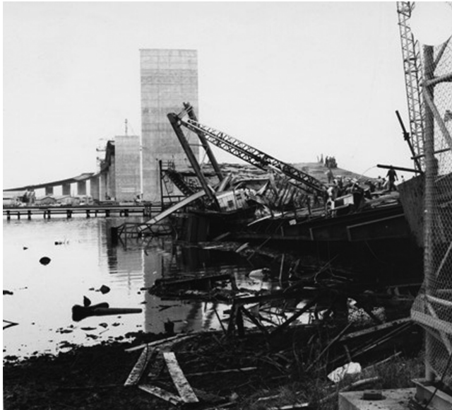
Figure 2.6 Westgate Bridge in Melbourne, just after the bridge collapse in 1970 (copyright courtesy of Westgate Bridge memorial committee).
