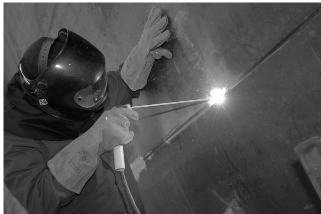
Figure 3.2 Manual metallic arc welding of a steel panel (© TWI).
