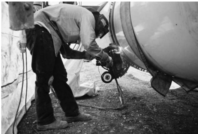
Figure 3.4 Mechanised welding of a gas pipeline girth weld, using a gas metal arc welding and a 'bug-on-band' system to ensure consistent welding (© TWI).
