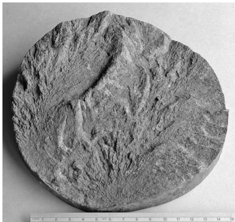
Figure 8.15 A corroded (rusty) failed bar showing evidence of river lines pointing to an initiation point at the bottom of the image, suggesting a brittle fracture has occurred (© TWI).
