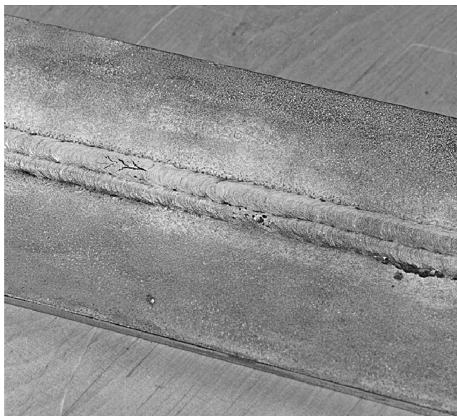
Figure 10.2 Chevron-shaped surface-breaking cracks detected in weld metal using dye-penetrant testing. The dye is usually dark red, exposed onto a background of a white developer to highlight any cracks found (© TWI).
