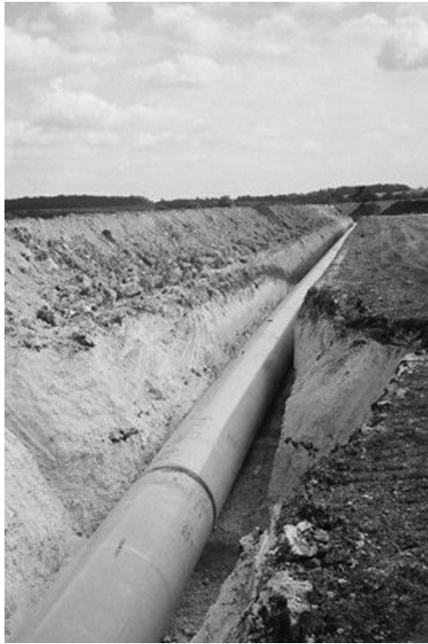
Figure 1.4 Girth weld in a gas transmission pipeline in the UK before being buried (© TWI).
