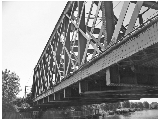
Figure 1.5 An example of a typical riveted construction railway bridge, crossing the river in Cambridge, UK (© TWI).
