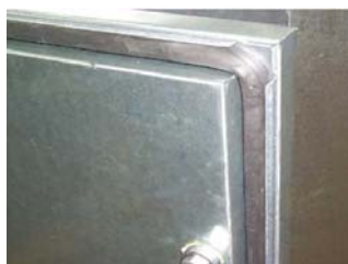
Mechanically fixed replaceable door seal
