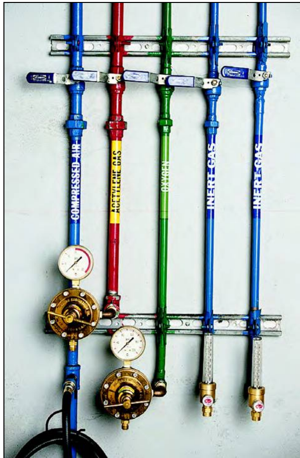
Figure 2.11—Acetylene and Oxygen Regulators and Inert Gas Flowmeters
