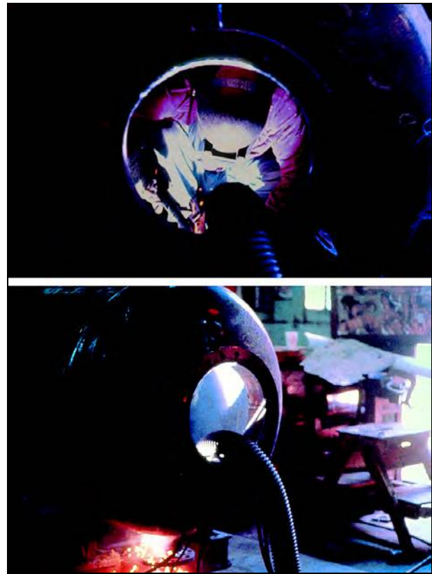
Figure 2.9—Welding in Confined Spaces
