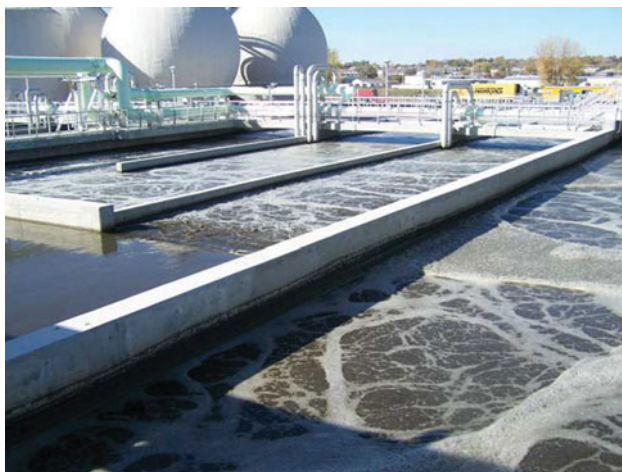
Figure 4.6 Aerobic basin with supplemental dissolved oxygen system (Reproduced with permission from © DDM Imagery).
