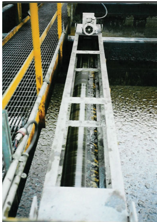
Figure 2.8 A rotary drum oil skimmer (Reproduced with permission from © Skim oil™, Inc.).
