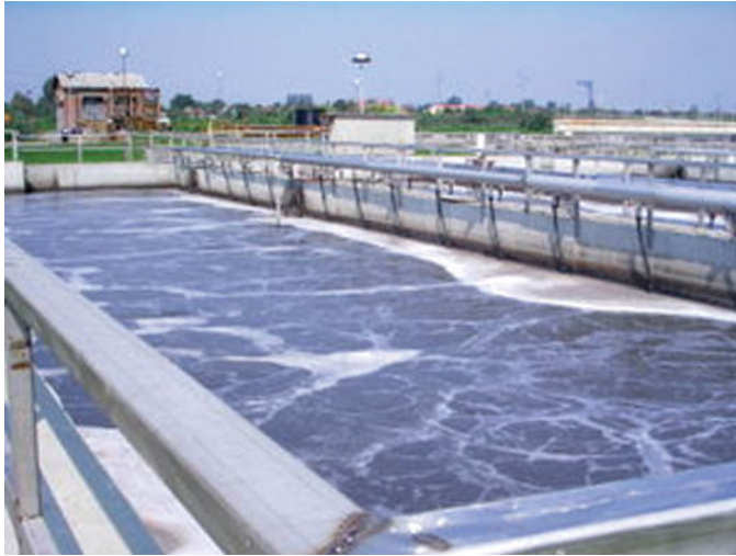
Figure 4.3 Aerobic basin (Reproduced with permission from © AECOM).
