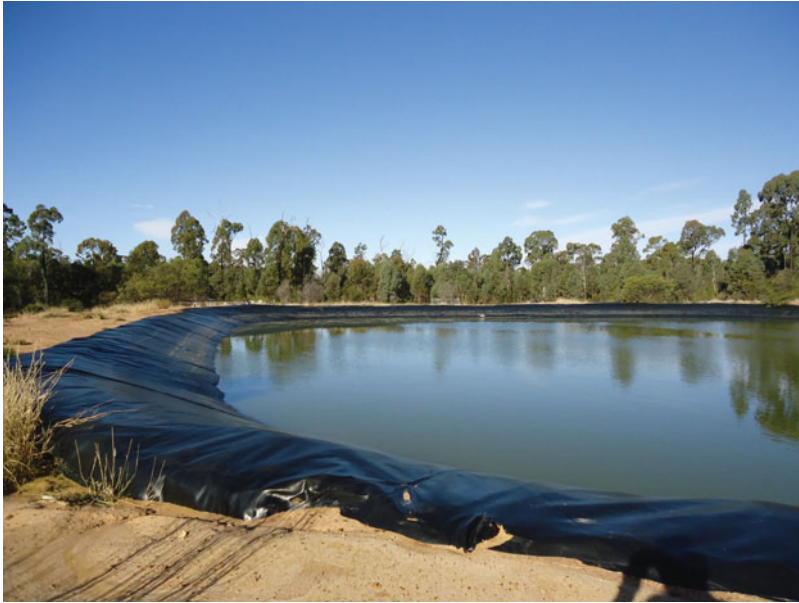
Figure 5.2 A holding pond at Woodview, west of Casino, used by a coal seam gas company to store wastewater (Reproduced with permission from © Green-left, NSW, Australia).
