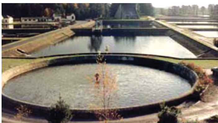
Figure 4.13 Sewage oxidation ponds (Reproduced with permission from © DDM Imagery).
