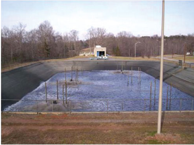
Figure 2.10 An equalization basin (Reproduced with permission from © Hickory wastewater treatment).
