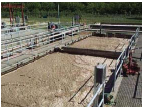
Figure 7.5 A sludge digester (Reproduced with permission from © DDM Imagery).
