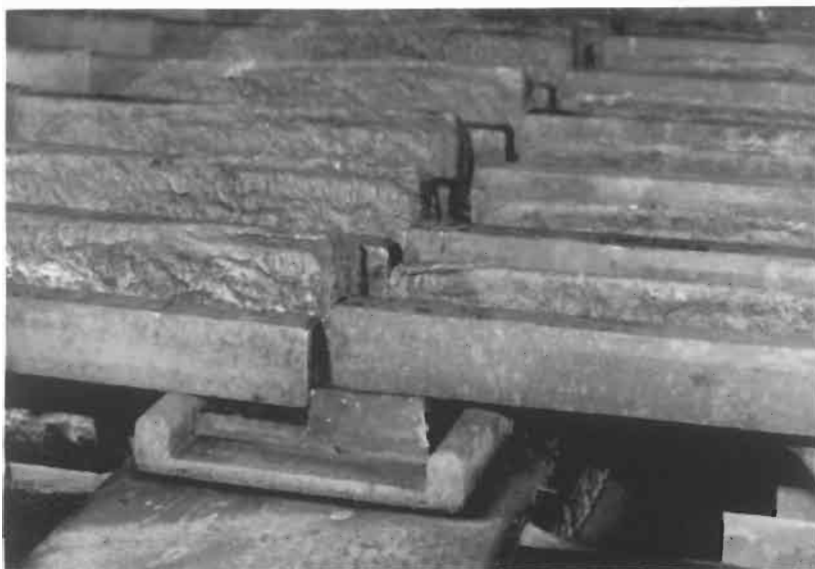
Fig. 16.2c. Anode-cathode connections in industrial electrorefinery (photograph courtesy R. Douglas Stern, Phelps Dodge Mining Company). The cathode in the left foreground rests on a copper conductor bar, the anode behind it on an insulator. The cathode in the right foreground rests on the insulator, the anode behind it on the copper conductor bar. Electric current passes:
