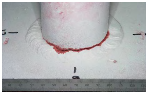
Crack found using dye penetrant inspection.
