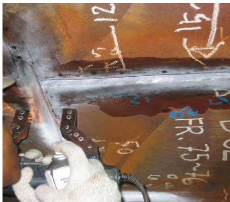
Magnetic particle inspection using a yoke.
