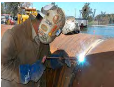
Examples of the MMA welding process
