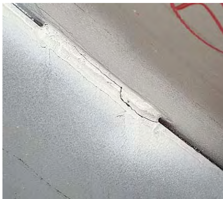
Crack found using magnetic particle inspection.
