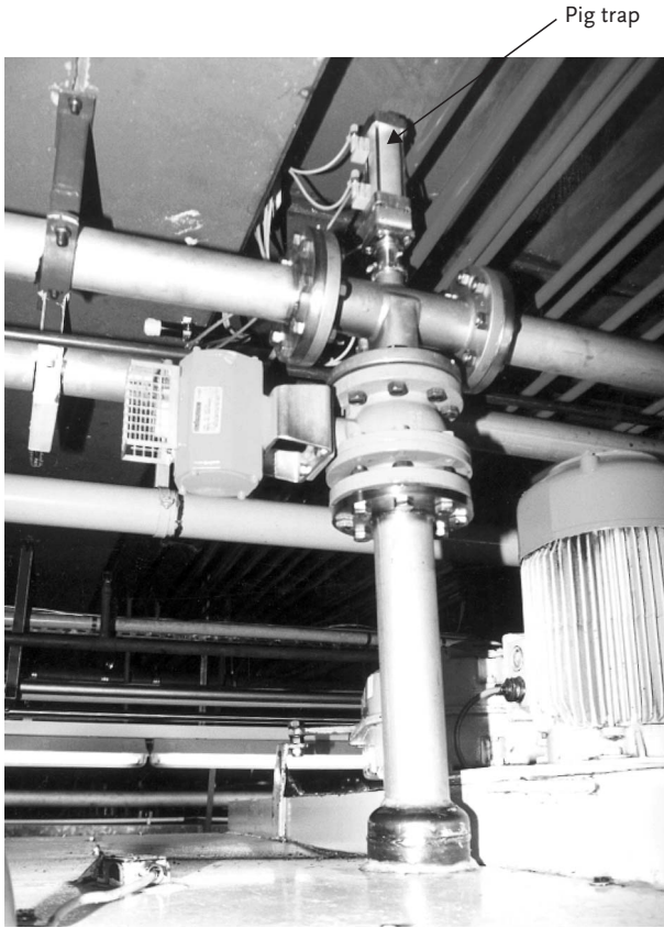
Fig. 4-11. Pig trap (I.S.T., Hamburg, Germany)
