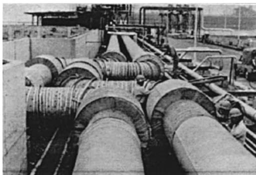
Figure 5.38 LPG Pipelines by Frothing-in-Place, [5.44].
