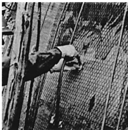
Figure 4.13(b) Frothing-in-Place Operation onto Tank Surface [4.54].
