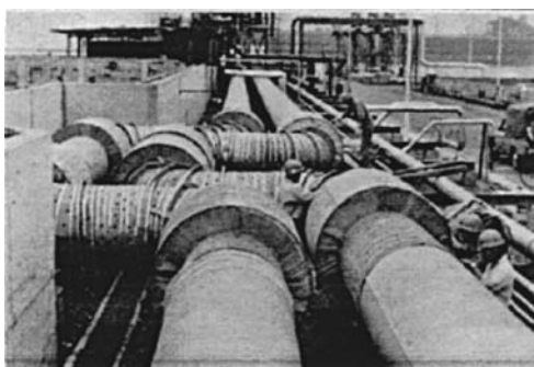
Figure 4.15 LNG Pipe Lines Insulated by Frothing-in-Place [4.54].
