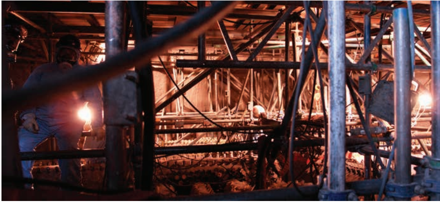
FIGURE 5.5 – Health and safety aspects are key issues for any shutdown
