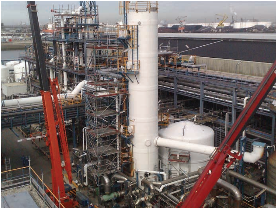
FIGURE 1.1 – A shutdown can be an extensive operation involving much equipment and many external personnel
