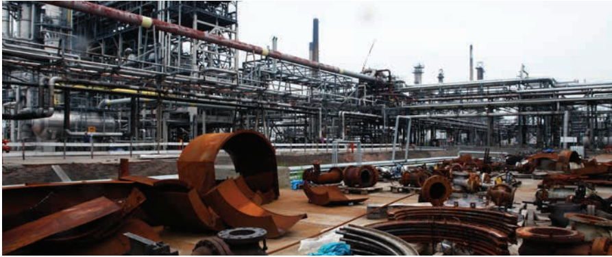
FIGURE 2.13 – Temporary storage of materials during shutdown
