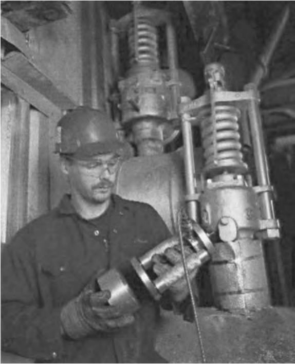
Figure 17.2 A mechanic performing safety valve maintenance. (Courtesy Mobile Valve Repair Ltd., Canada.)
