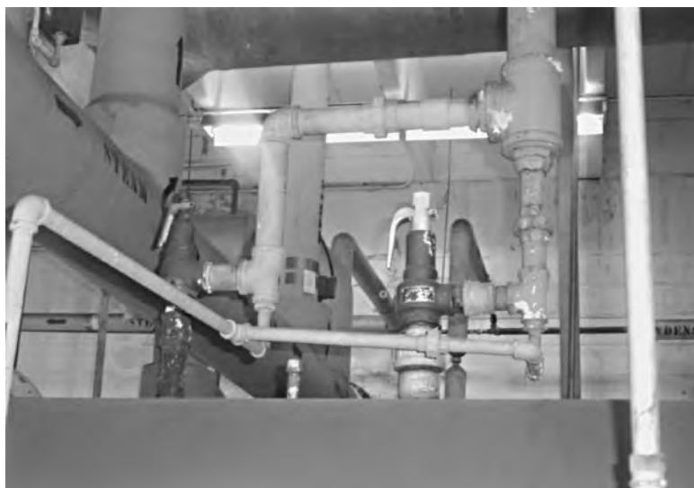
Figure 15.14 Safety valves installed on a power boiler.
