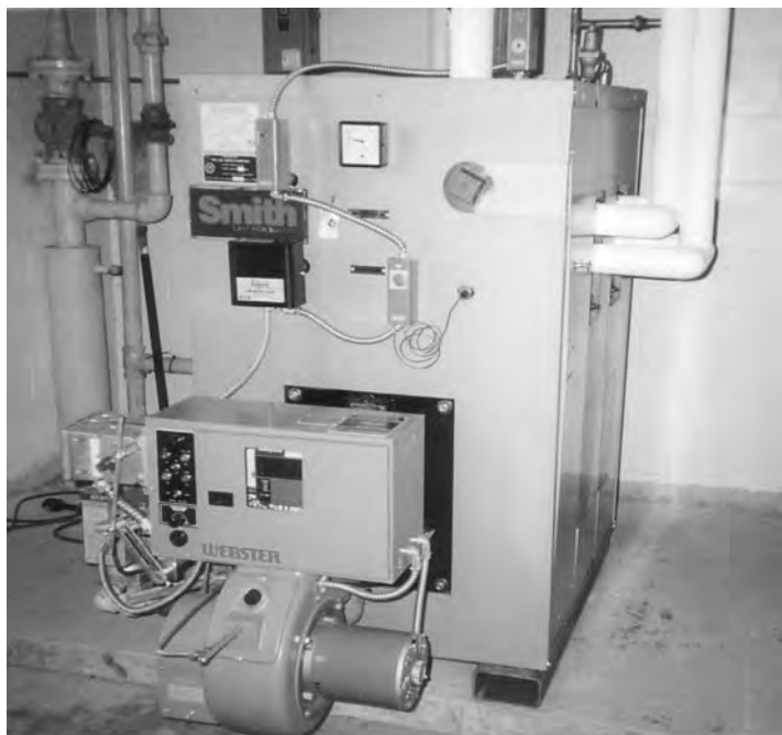
Figure 10.1 A typical low-pressure steam boiler.
