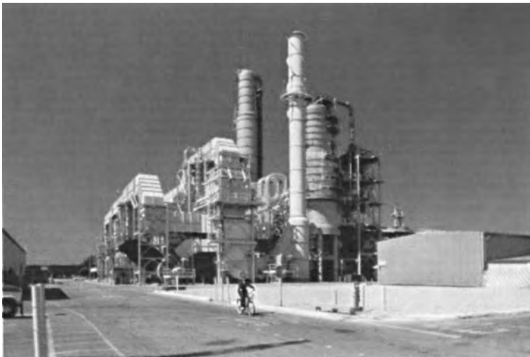
Figure 14.2 Crude unit of a refinery.
