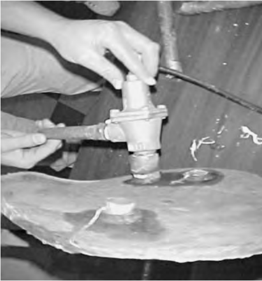
Figure 1.3 T&P pressure relief valve after explosion.
