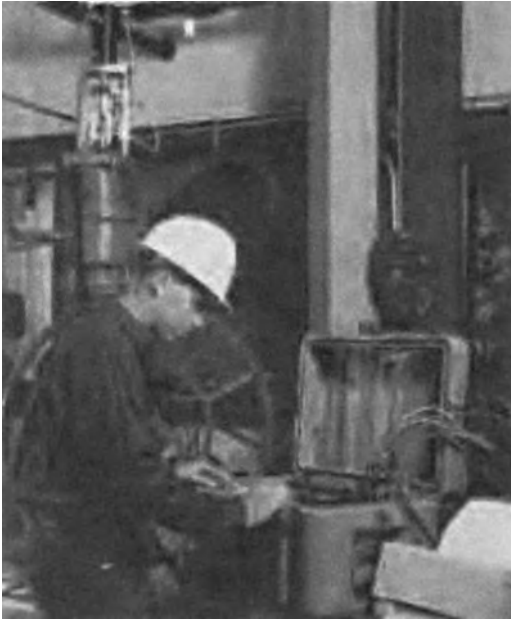
Figure 18.3 In-line valve testing. (Courtesy B & HES, Inc.)
