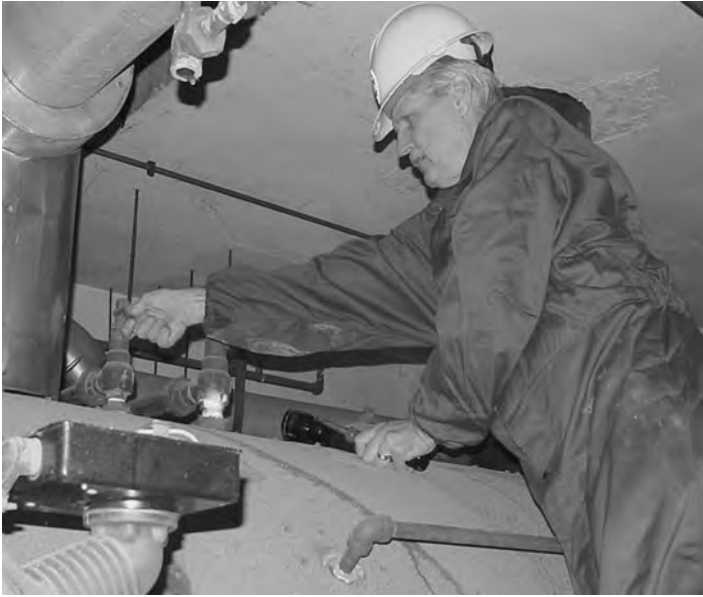
Figure 18.4 Safety valve inspection by an AI.
