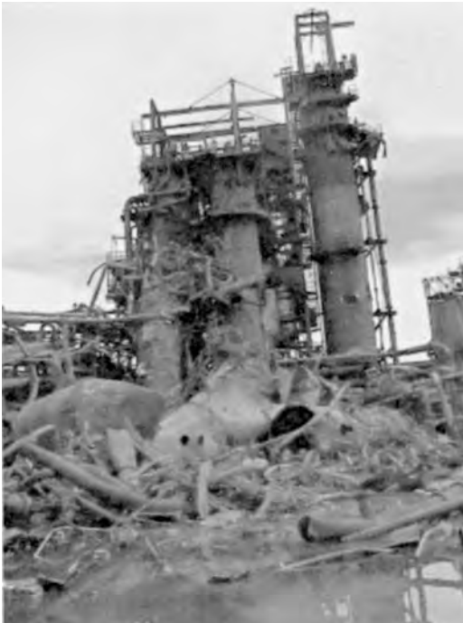
Figure 1.4 Digester system explosion in Kaiser Alumina Plant. (Courtesy Federal Mine Safety and Health Administration.)
