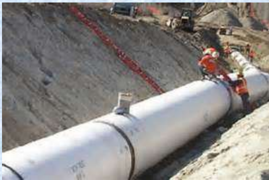
Weld on Pipe
