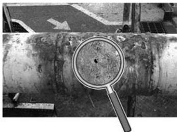
Figure 6.9 Corrosion under insulation (CUI)
