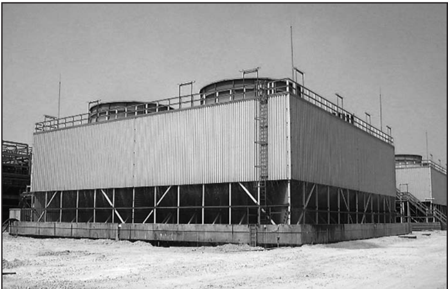
Figure 7–17 Typical arrangement of a wet-cell cooling tower
