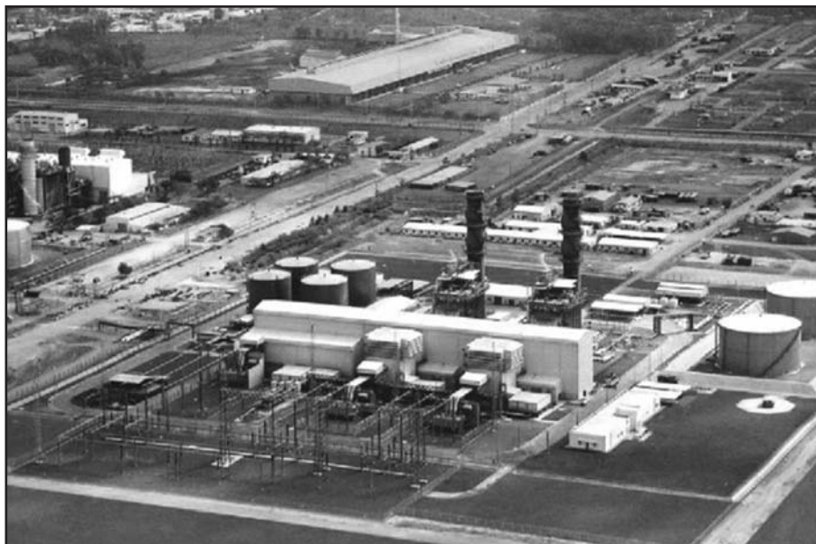
Figure 14–6 View of the Phu My 3 combined-cycle power plant
