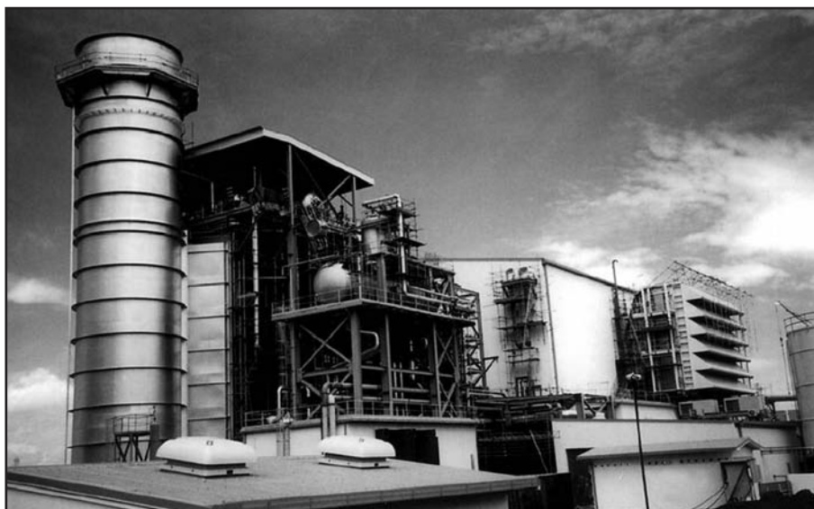
Figure 14–1 View of Taranaki combined-cycle plant
