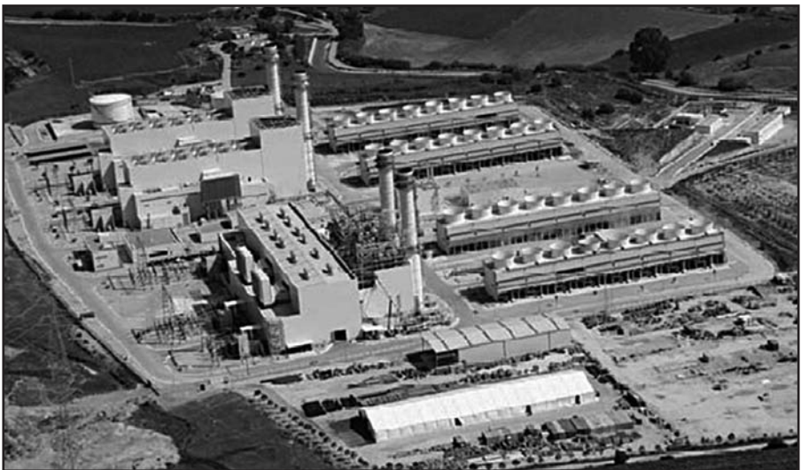
Figure 14–12 View of the Arcos combined-cycle power plant
