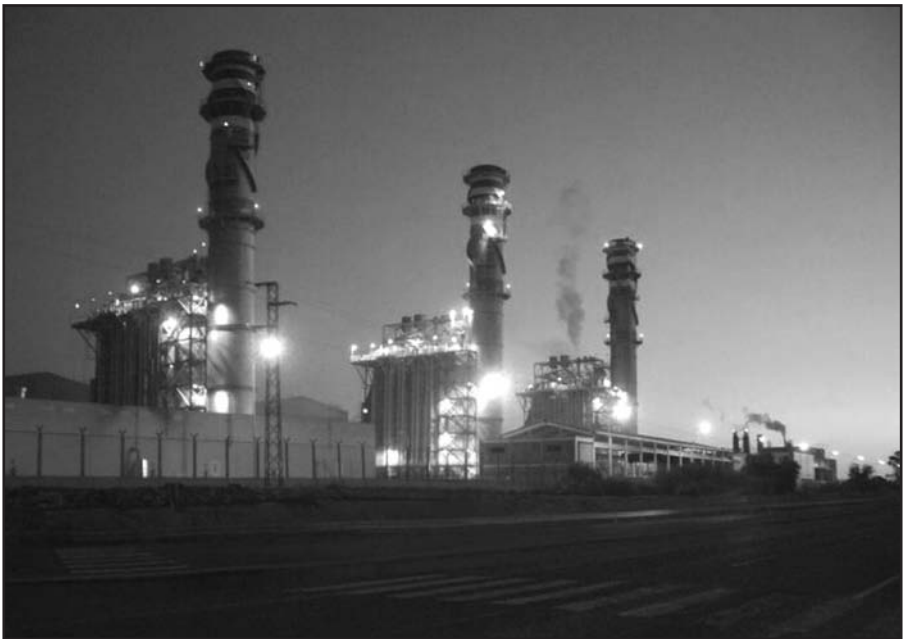
Figure 14–9 View of the Palos de la Frontera combined-cycle power plant
